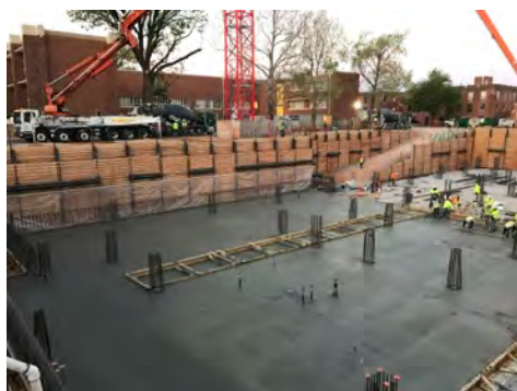
Foundation of Lin Hall. Construction will be concluded by the summer of 2018.
